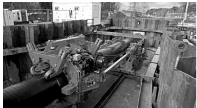
Picture 3. Cylinder based pipe thruster produced by the German company Herrenknecht since 2006
